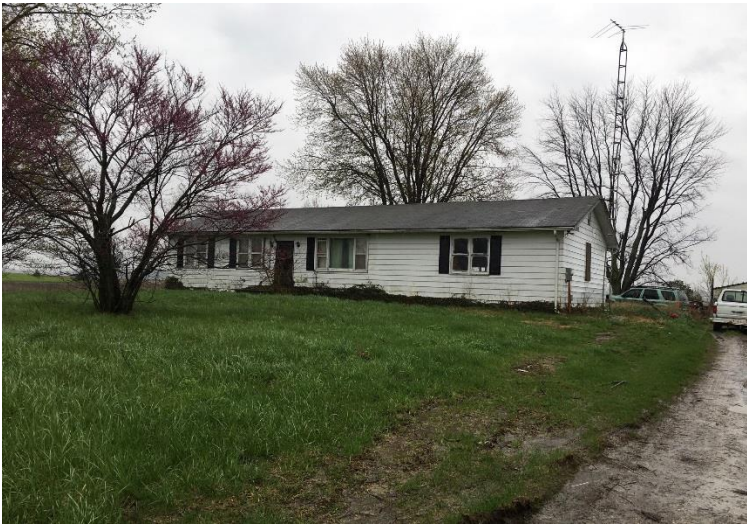
3101 Monnett New Winchester Rd Caledonia
